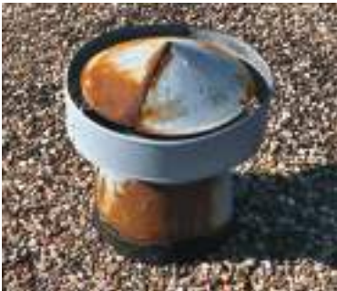
Rust Damaged Roof Fixture
