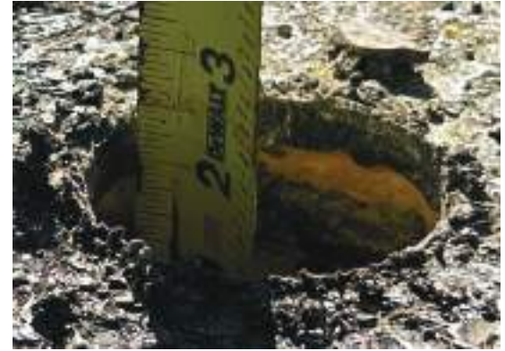
Approx. roof material depth is 2.5 inches
