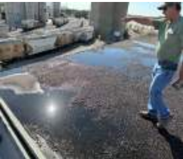
Perimeter Rainwater Ponding
