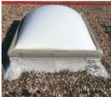
Skylight Curb Repairs
