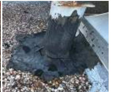
A/C Footer Penetration Repairs
